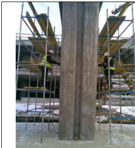
Fig. 1. Ultrasonic testing to determine the concrete strength in monolithic structure
